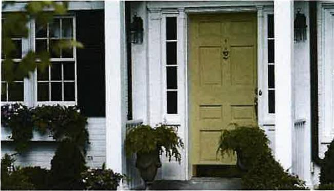
**Doors:** Shall be painted or stained wood, fiberglass or steel with raised panel profiles. Transoms and sidelights shall have true divided lights or simulated divided lights with mullions. Garage doors shall be wood, fiberglass, or aluminum and shall be painted or stained.
